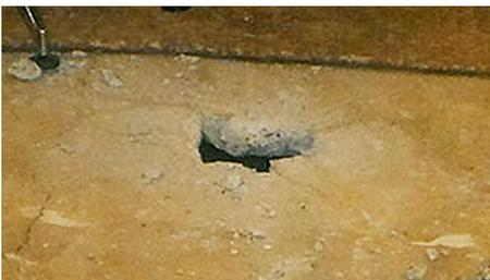
Hole in the concrete floor as a result of the burst pipe.
